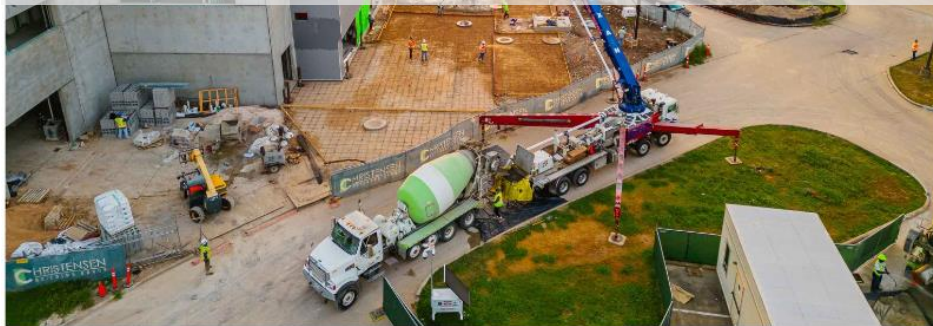
OPUS SCM concrete for the Porsche Sugar Land pour batched, placed, and finished like conventional mixes.
